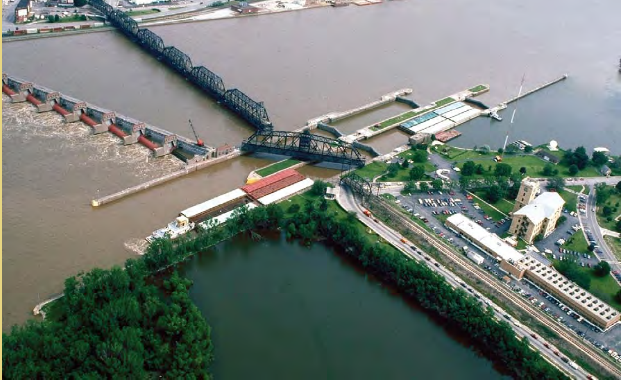
Mississippi River Lock and Dam No. 15 at Rock Island, IL (bottom) and Davenport, IA (top), with the Government Bridge over the river. Adjacent to the U.S. Army's Rock Island Arsenal, an active installation and a National Historic Landmark.
